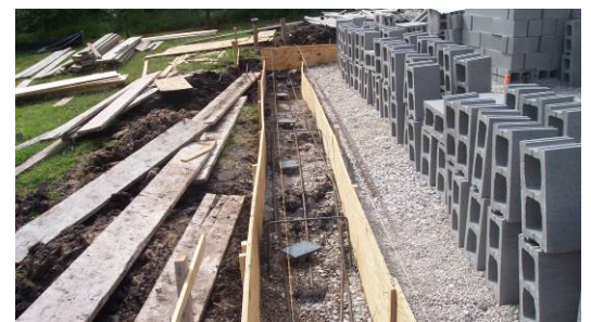
Foundation under construction
