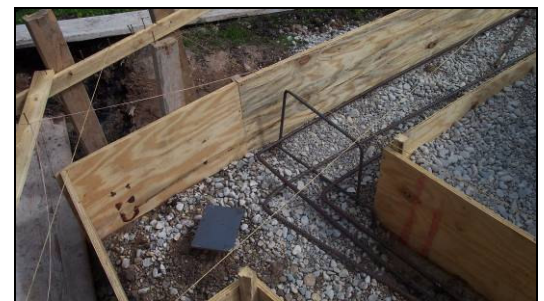
Foundation under construction
